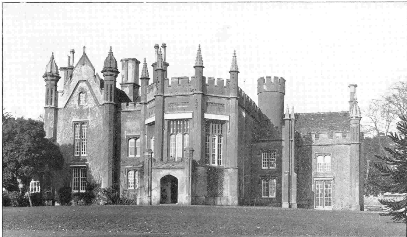
CROWE HALL, STUTTON (South View).
