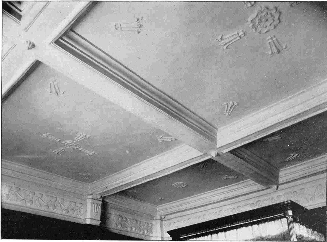
CEILING IN STUTTON HALL.
